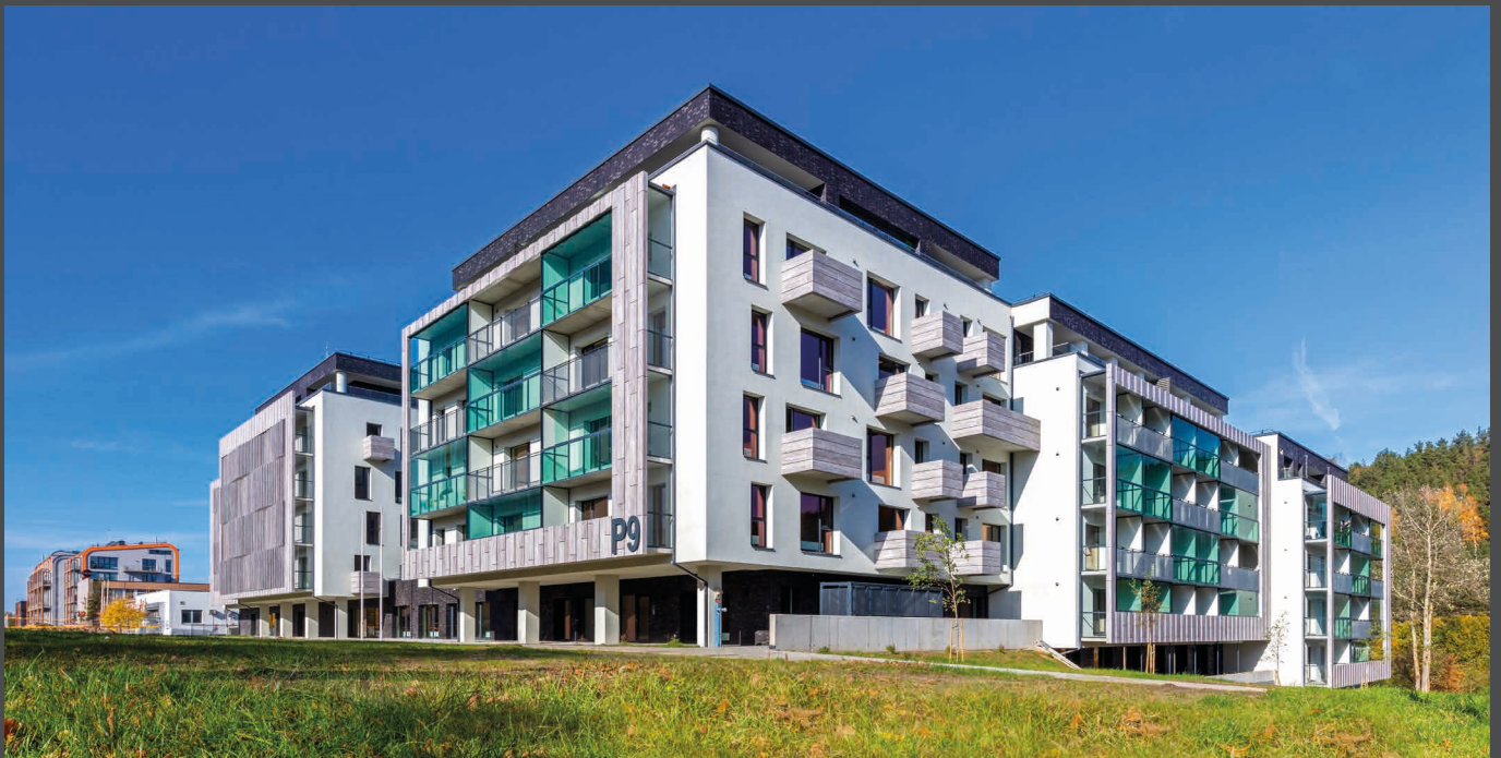
P9 Paplajus apartments, Lithuania | Material: ALUCOBOND® PLUS legno Antique Pine | Architect: 313 Architects | Fabricator: LR group | Installer: Lakede | © Evaldas Lasys
